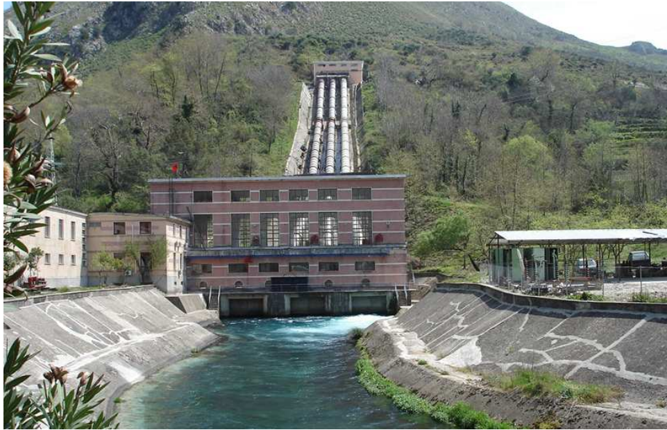
Small Hydro-Power Plant in Albania
