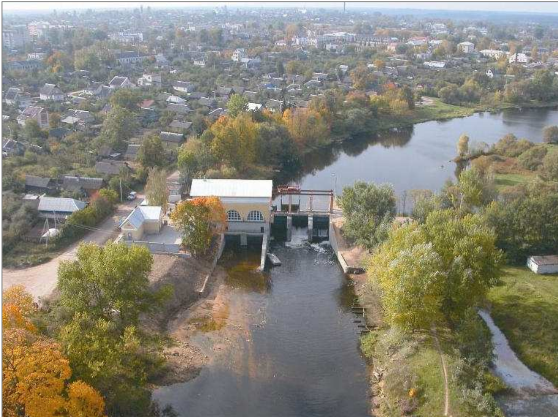
Lepel Small Hydropower Plant (Vitebsk Oblast)
