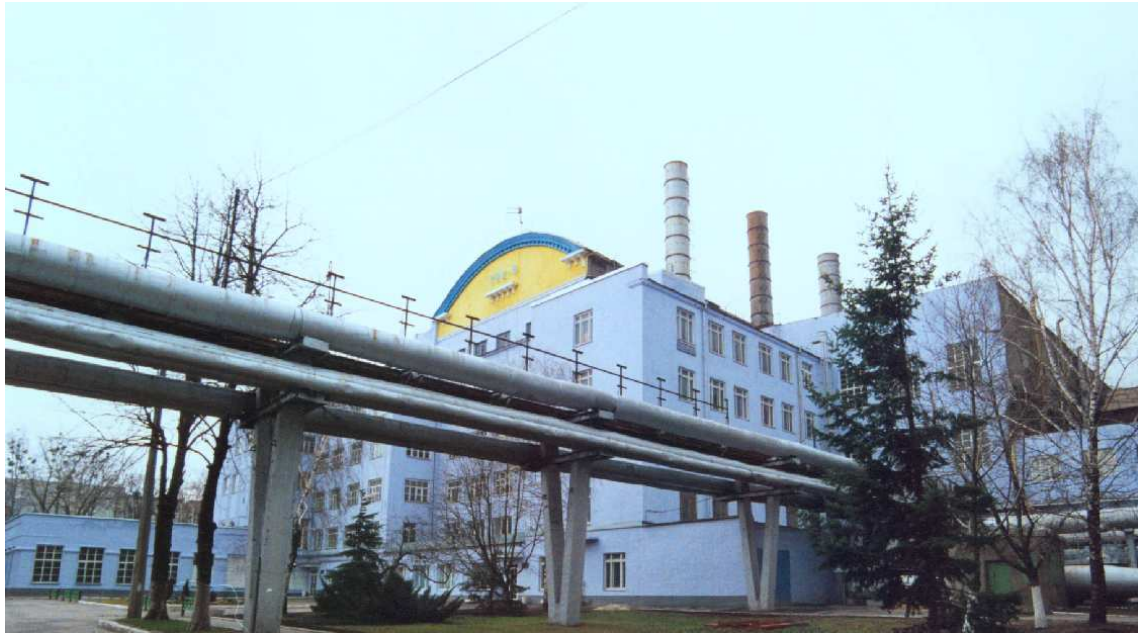
Kharkiv Combined Heat and Power Plant (CHP-3)
