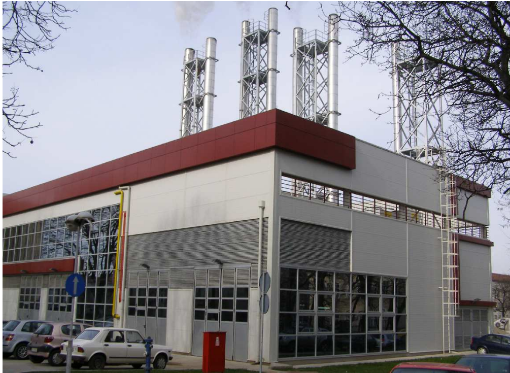
Co-generation energy facility in the Clinical Center of Serbia
