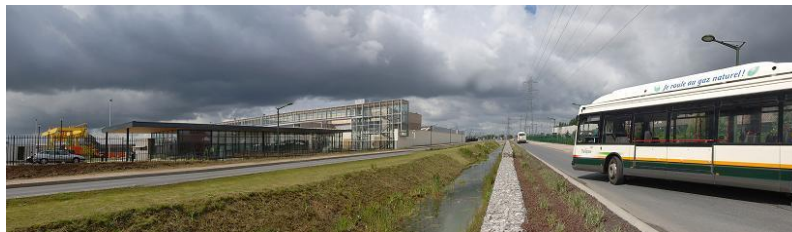
The road between the Organic Recovery Center and the bus depot over the dedicated pipeline
