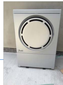
(e.g. Air source heat pump)
