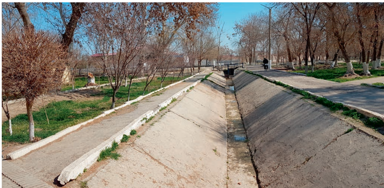
Photo 3: Stormwater channel in Samonids Park, Bukhara City
