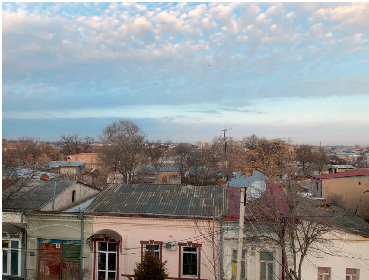
Photo 17: Roofing with corrugated asbestos sheets, Samarkand City
