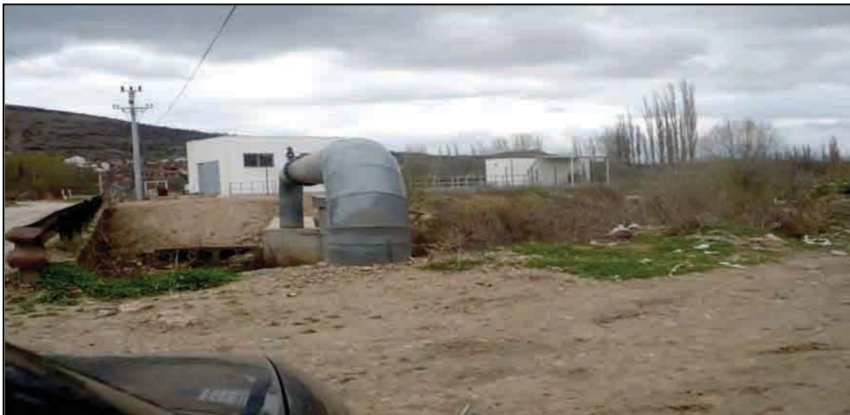
Image 2. Main collector with pump station
