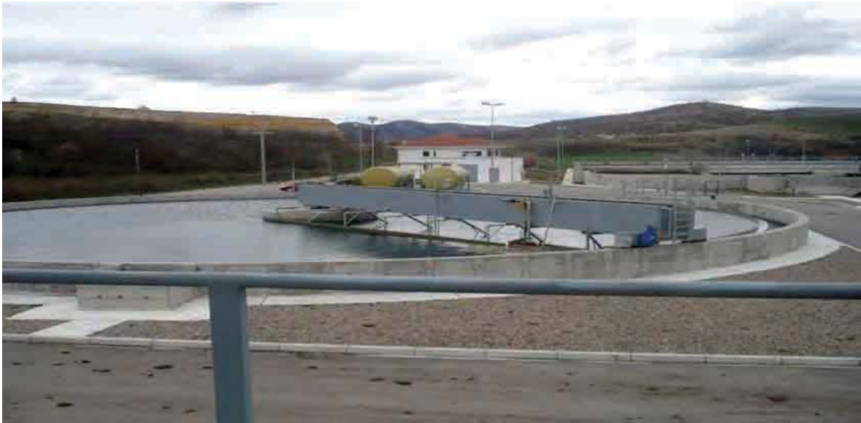
Image 1. Urban waste water treatment plant – Dobrosane
