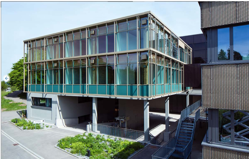
Fig. 1 The House of Natural Resources on the ETH Zurich's Höggerberg campus may appear small and unremarkable from outside, however it contains numerous innovative and pioneering wood-based features.
