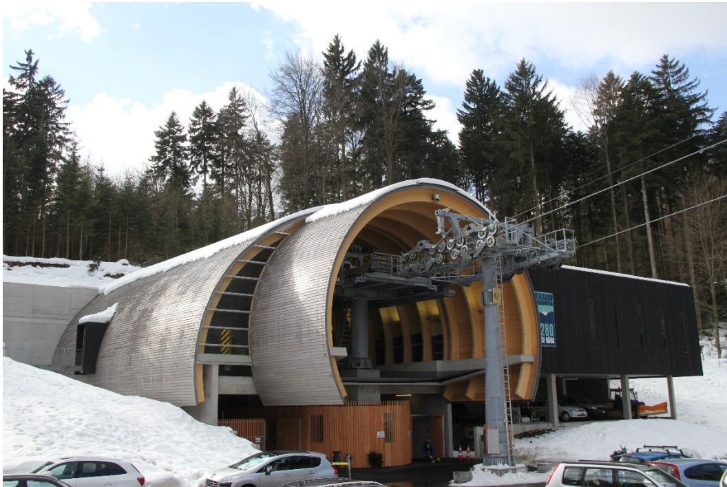
Fig. 4 – Weissenstein Cableway valley station (Image source: Guido Kummer + Partner Architekten, Solothurn)
