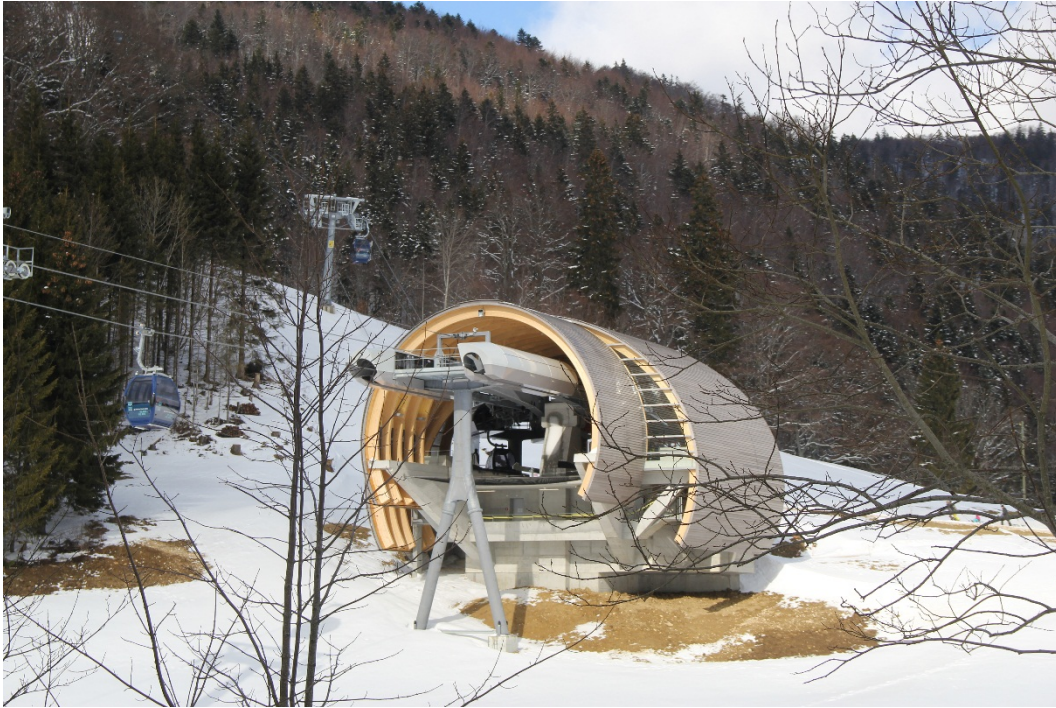
Fig. 5 – Weissenstein Cableway middle station (Image source: Guido Kummer + Partner Architekten, Solothurn)
