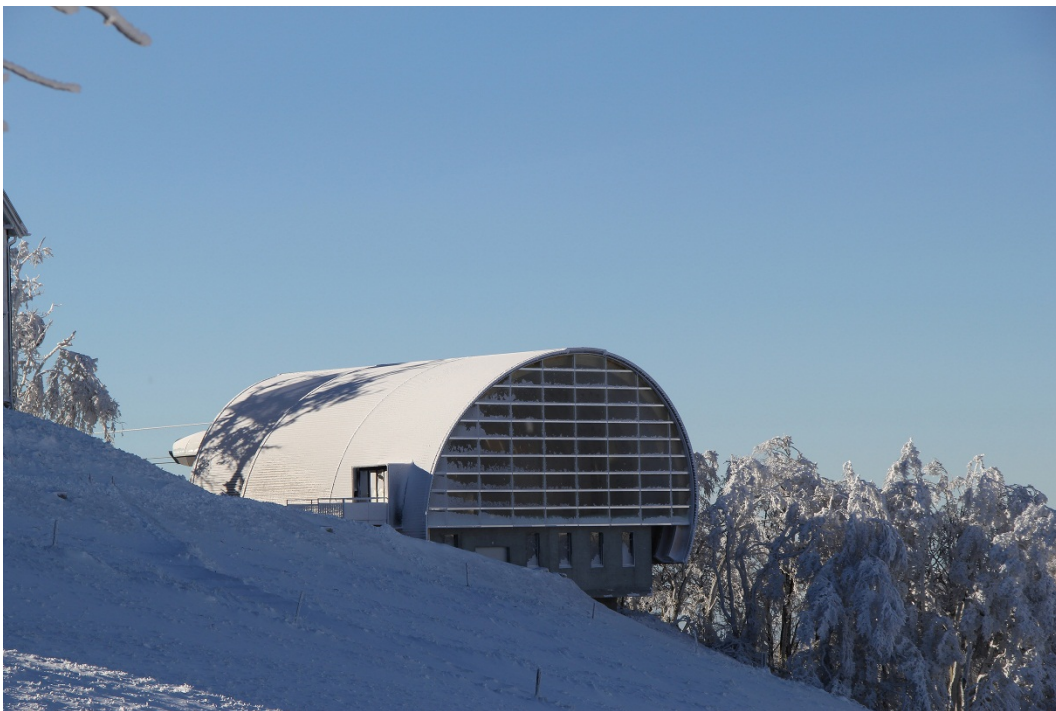
Fig. 6 – Weissenstein Cableway mountain station (Image source: Guido Kummer + Partner Architekten, Solothurn)
