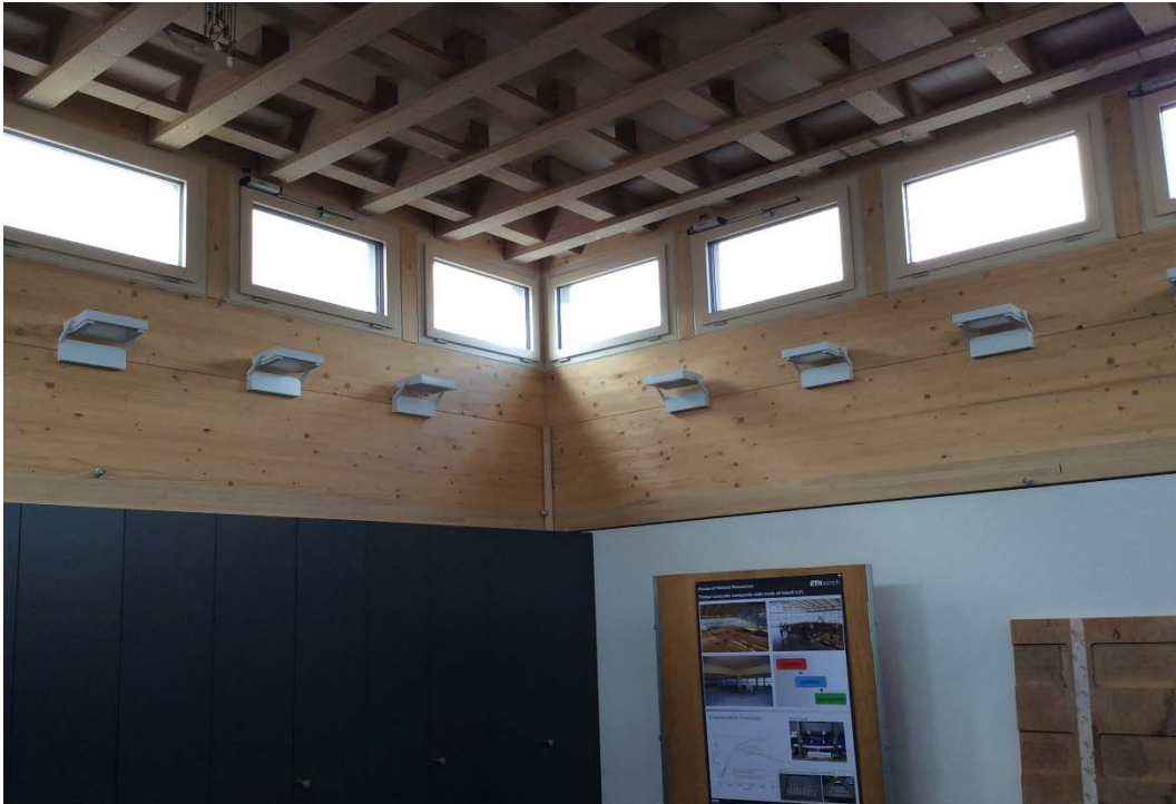
Fig. 2 The beech slab with its crossing beechwood lamellas is the first of its kind in the world. (Image source: Eduard J. Belser )
