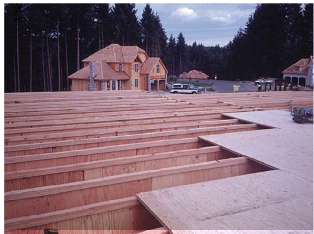
I-beams used for raised residential floors
