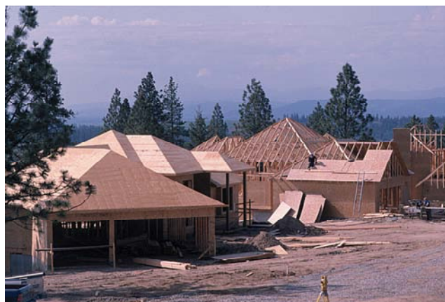
FIGURE 3.2.1 US residential construction
