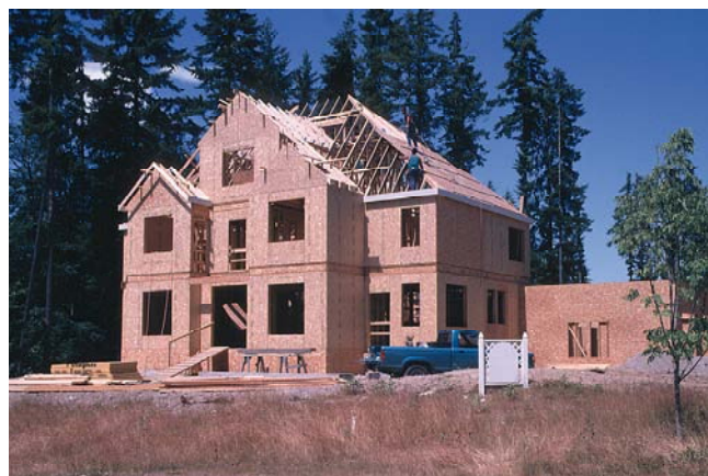
FIGURE 7.4.1 OSB in North American residential construction
