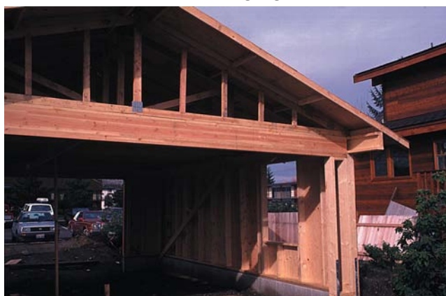
Glulam beam used for garage door header
