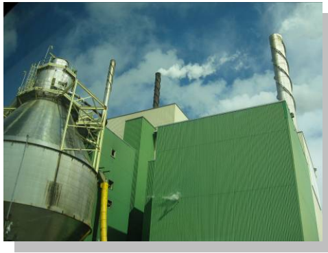
Mill-level environmental improvements
