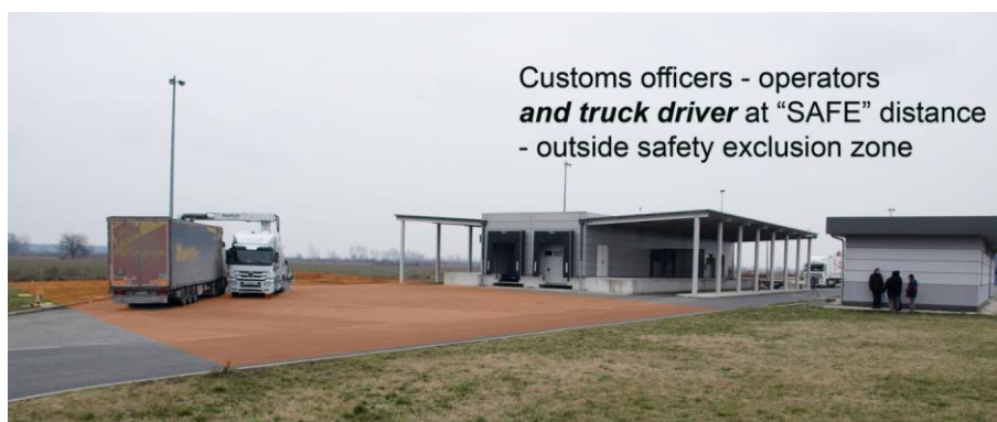
Picture 7 - LINAC exclusion zone showing scanner and scanned truck and position of the operators and driver outside the exclusion zone, real observed situation.
