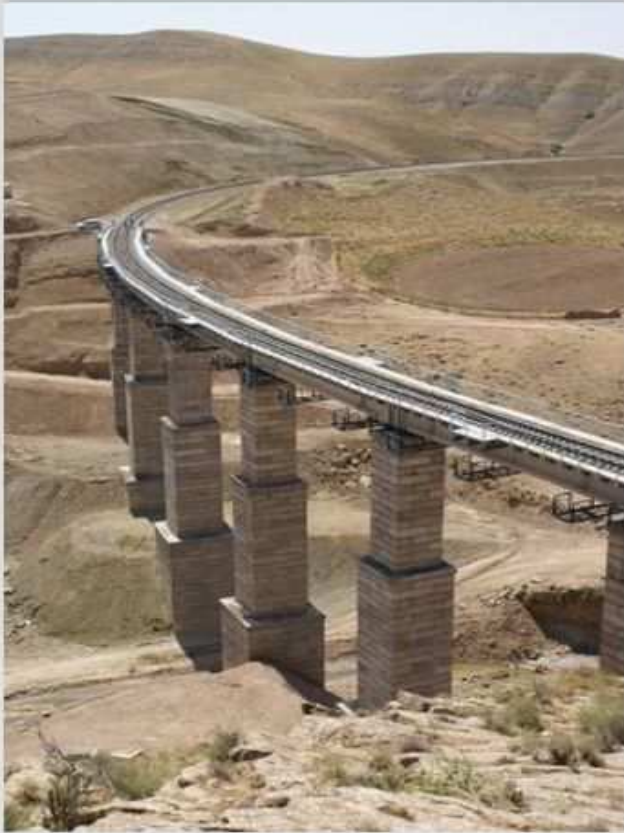
Railway bridge with iron superstructures
