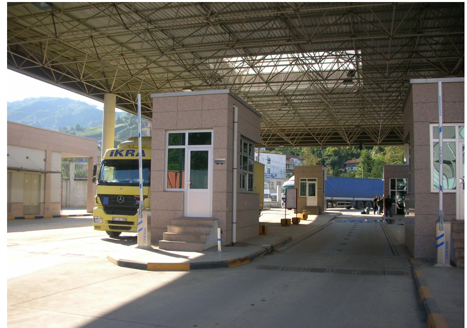
Good practice BCP asset management: several truck lanes each with one booth built to the truck window height
