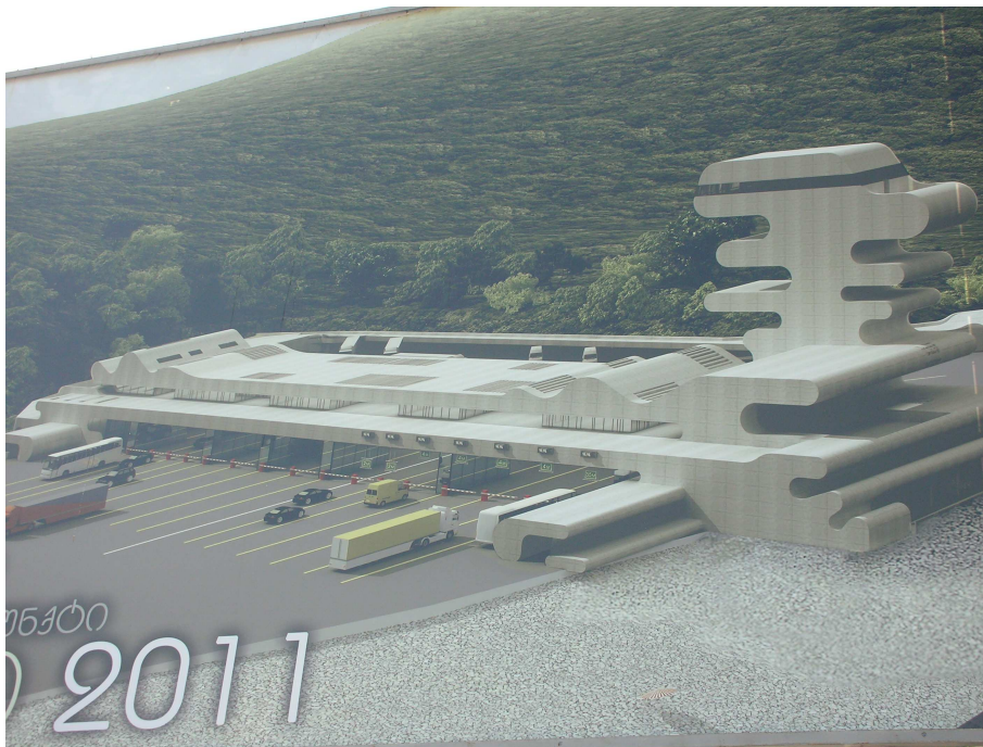
Georgia-Turkey Sarpi BCP: 15 traffic lanes with segregated truck lanes and fast track lanes
