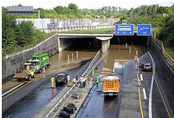
Inundation of tunnels
