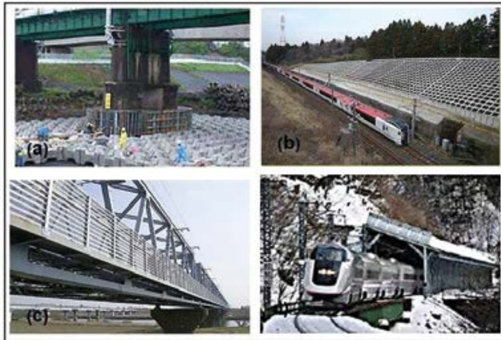
Figure 56 (a) Scouring protection (b) Slope reinforcement (c) Windbreak fence/screen and (d) anti-avalanche facilities.
