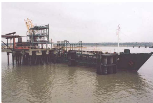
Figure 1 Barge loading operation at a petroleum terminal.
