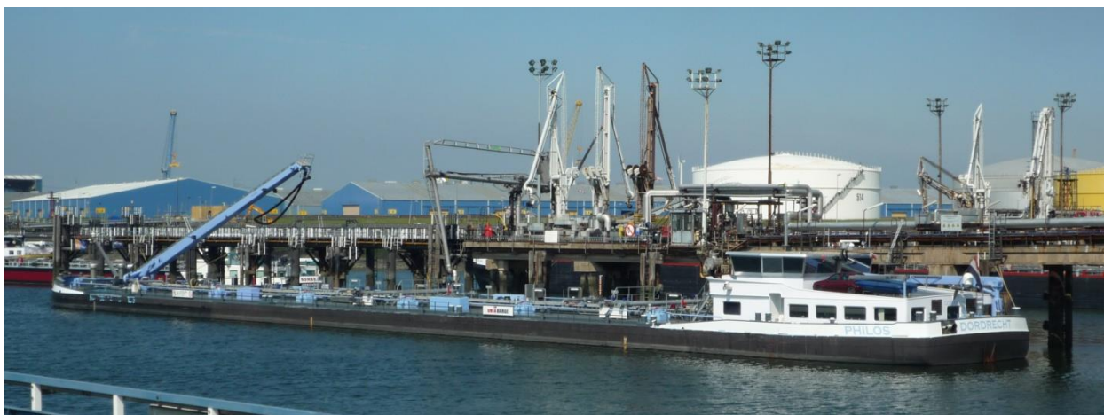
Figure 4 Photograph of a typical barge loading facility
