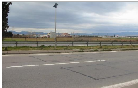
Continuous Permanent Traffic Counter & Classifier
