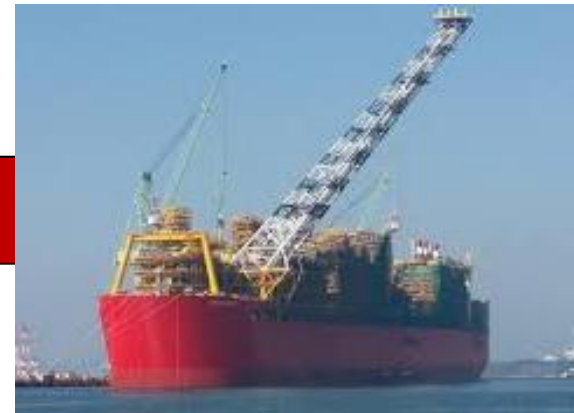
2017 : Shell Prelude FLNG – 326 000 m 3 (10 tanks)
