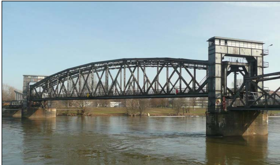
Bridge at the river Elbe
