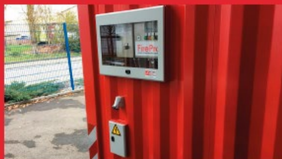
Integrated FirePro fire alarm and Aerosol extinguishing system
