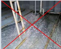
During loading of many flammable liquids in tanks, there is the risk of electrostatic accumulation and discharge in the form of a spark.
