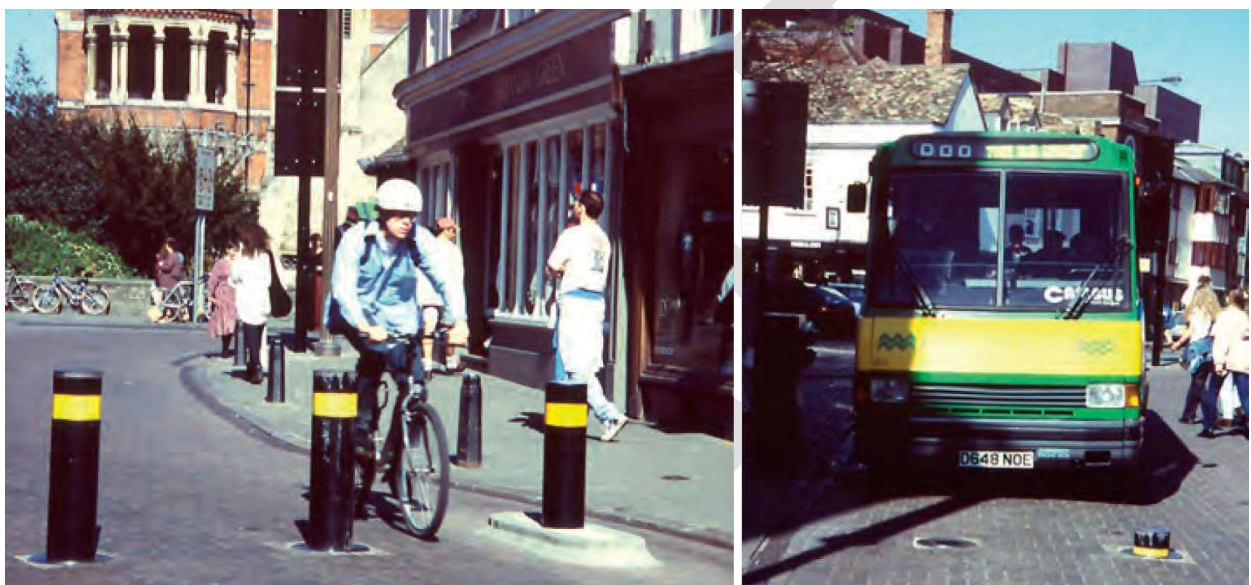
Figure 3.27. In Cambridge (UK), bollards serve to block entrance into the city centre for all modes of transport except PT and service vehicles
