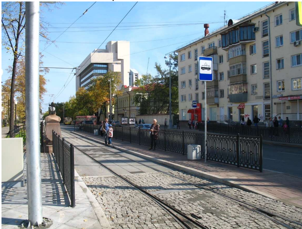
Figure 3.40. Installation of a tram platform on Lenin Avenue in Yekaterinburg (Russia)
