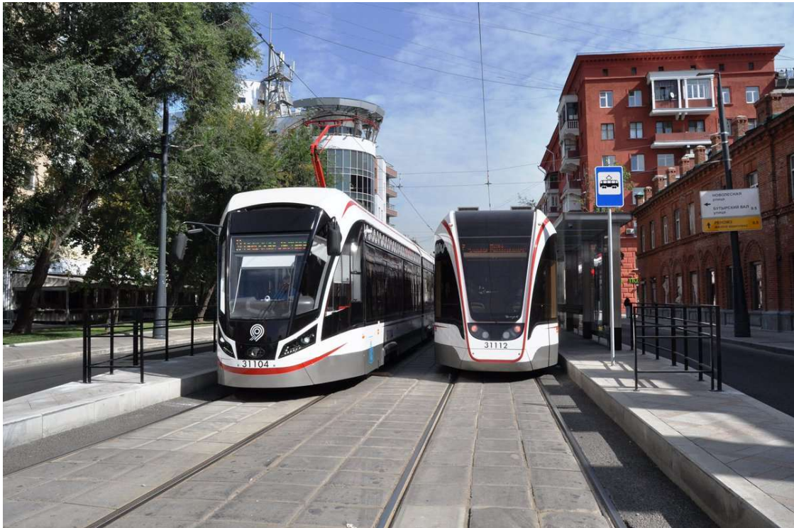
Figure 3.39. A tram line efficiently isolated with a curb on the Boulevard Ring in Moscow (Russia)
