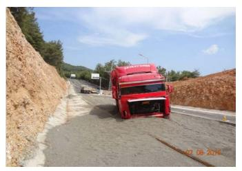
Truck escape ramps are constructed for accommodating out-of-control trucks on long steep downgrades.
