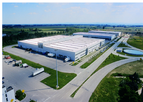
Large-sized warehouses (for logistic activities)
