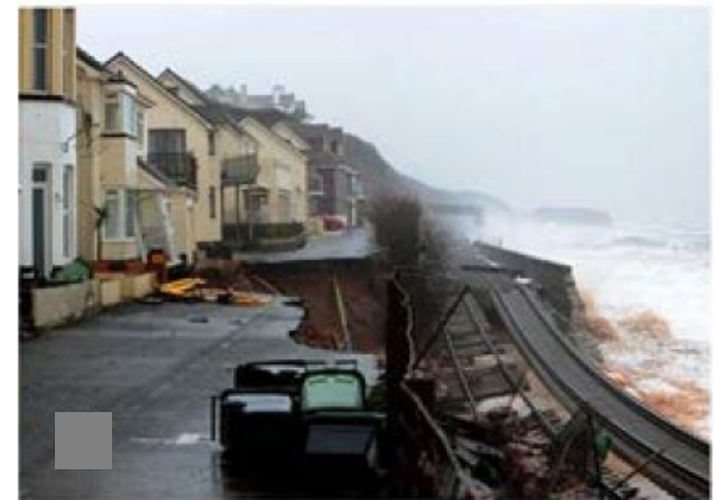
Storm destruction of the coastal railway in SW England (2013)
