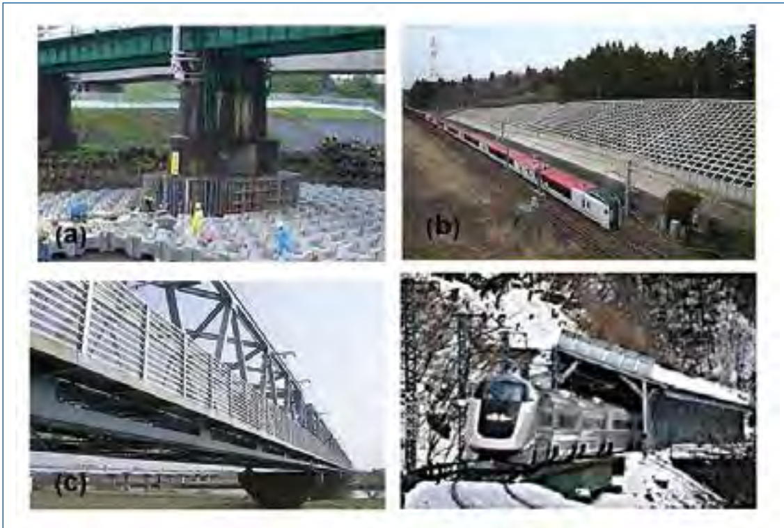
Figure 56 (a) Scouring protection (b) Slope reinforcement (c) Windbreak fence/screen and (d) anti-avalanche facilities.
