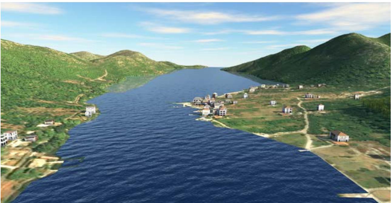
Figure 22 Existing conditions in project space
