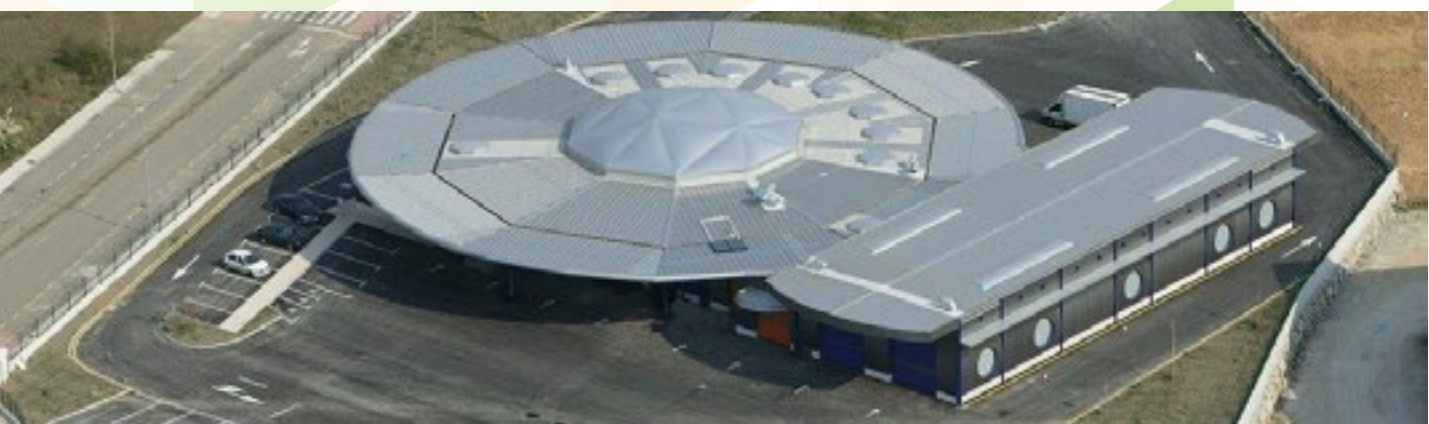
Not all PTI centres have a rectangular shape © Picture courtesy of itvasa of its facilities
