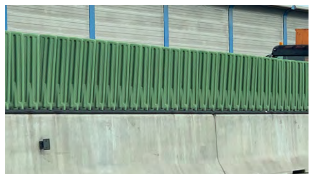
Figure 13: Anti-dazzle screens mounted on concrete barrier
