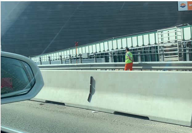
Figure 9: Examples of concrete (left) and steel (right) safety barriers
