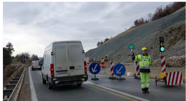
Figure 8: Traffic lights regulation in road work zones
