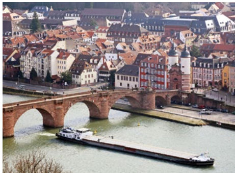
The Neckar in Heidelberg (Germany).
