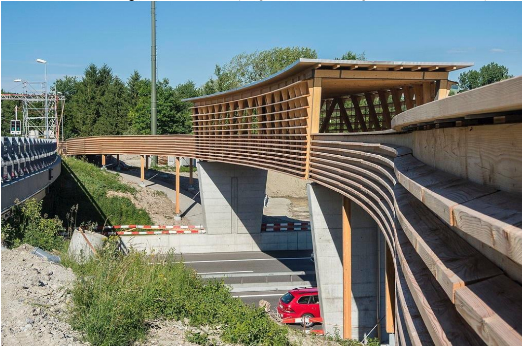
Fig. 10: Cycling and pedestrian bridge over the A6 motorway access road at Rubigen, canton of Bern: View from the west.(Image source: Emch & Berger, Willy Vogelsang)
