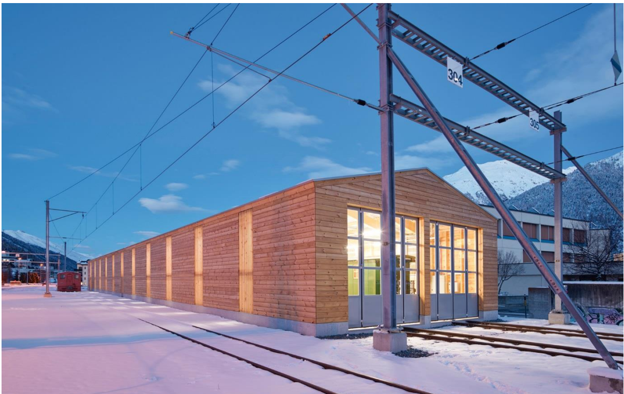
Fig. 1 and cover picture Shed for historical rolling stock of the Rhaetian Railway at Samedan (Image source: Brassler Architekten, Samedan GR)
