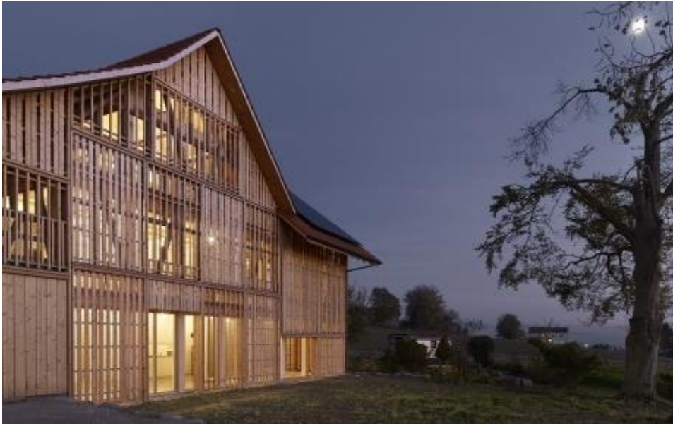
Fig. 12 Conversion of an old barn into a residential dwelling in the Dingenhart village conservation area, Frauenfeld, canton of Thurgau. The external look of an old barn is maintained in accordance with the conservation criteria. (Image source: Prix Lignum)
