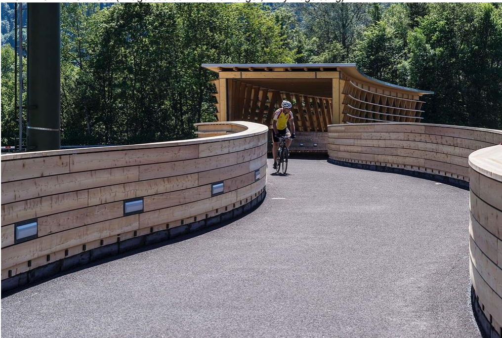
Fig. 11: Cycling and pedestrian bridge over the A6 motorway acces road at Rubigen, canton of Bern: Covered central part of the bridge crossing the motorway. (Image source: Emch & Berger, Willy Vogelsang)
