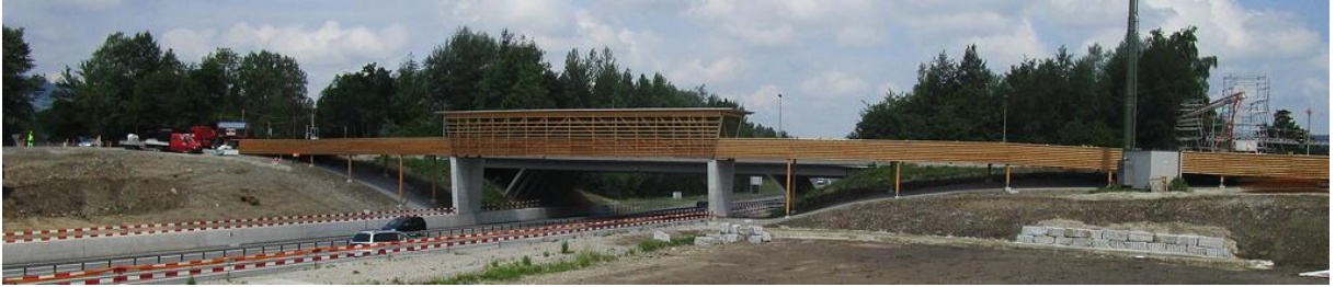
Fig. 9 Cycling and pedestrian bridge over the A6 motorway access road at Rubigen, canton of Bern; View of the entire bridge from the south. (Image source: Emch&Berger, Jean-Pascal Ammann)
