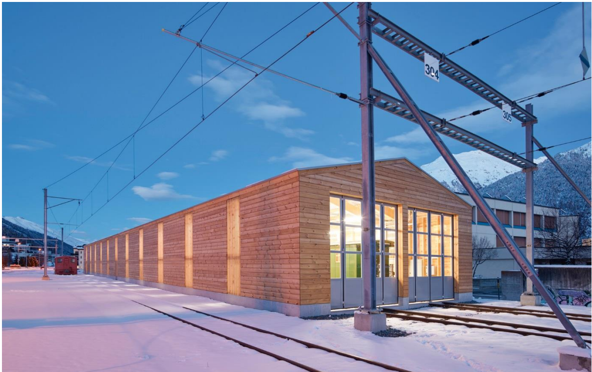
Shed for historical rolling stock of the Rhaetian Railway at Samedan (image source: Brasse Architekten, Samedan)
