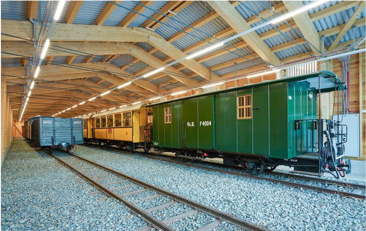
Fig. 2 Shed for historical rolling stock of the Rhaetian Railway at Samedan (Image source: Brasser Architekten, Samedan GR)
