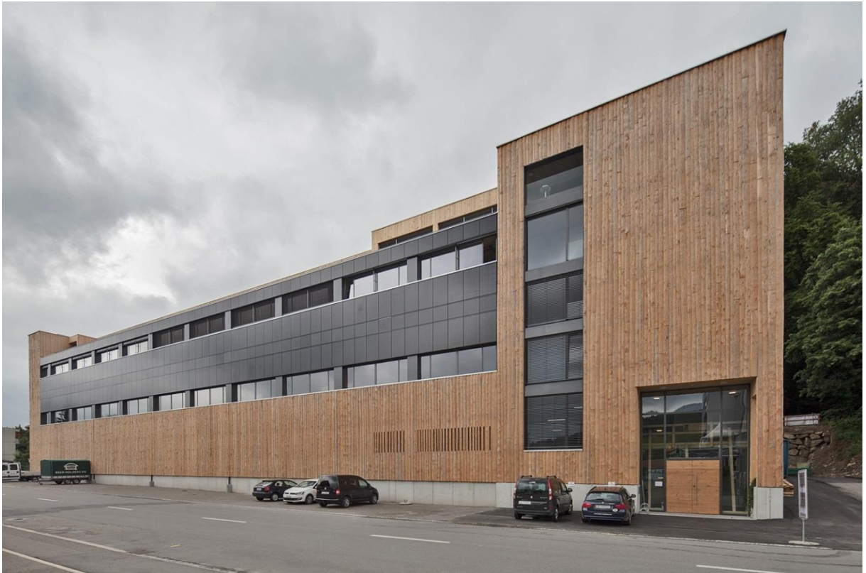
Fig. 3 "FachWerk" building including production facility, offices and residential units. The façade is fitted with solar panels (Image source: Beer Holzbau AG, Ostermundigen BE)
