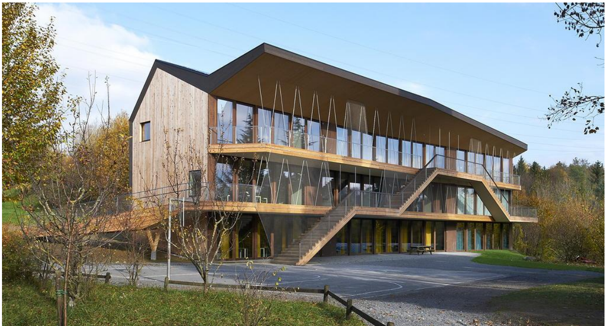
Fig. 7 Bois-Genoud Steiner School, Crissier, canton of Vaud: The cantilevered roof and terraces provide protection from the sun in the summer and facilitates solar gain winter. (Image source: LOCALARCHITETURE, Lausanne VD)
