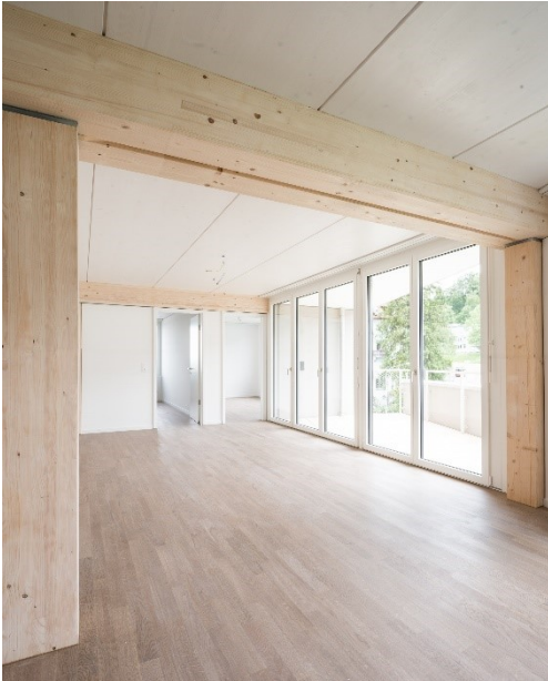
Fig. 6 Five-storey apartment block on existing semi-basement, the supporting structure influences the inside space (Image source: Till Forner, Zurich)
