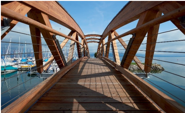
Fig. 22 Pedestrian and cycle path at the marina in Portalban, FR. (Image source: Prix Lignum)
