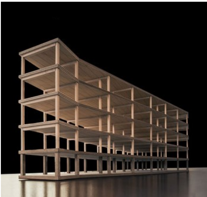
Fig. 5 Five-storey apartment block on existing semi-basement, model of the supporting structure (Image source: Till Former, Zurich)
