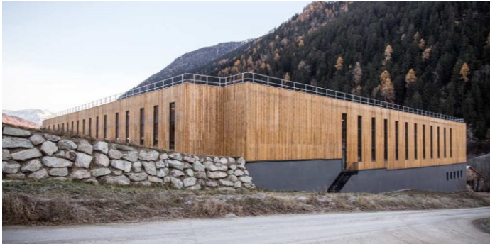
Fig. 7 Addition of storeys to warehouse and production hall for building material supplier LICO, Müstair in the canton of Graubünden and café. (Image source: Foto Martin Pinggera)
