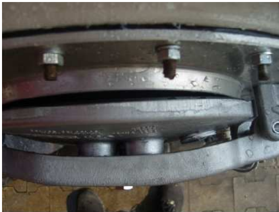
Picture 3: Failing filling hole cover after the test
